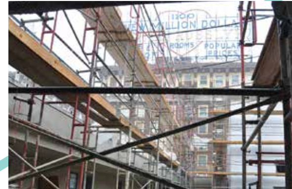
The New Genesis under construction.
